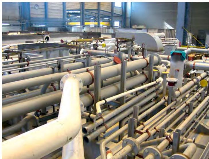
Figure 2. Prefabricated piping modules assembled in a workshop
