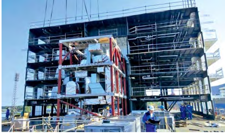
Figure 3. AC module being lifted and installed
